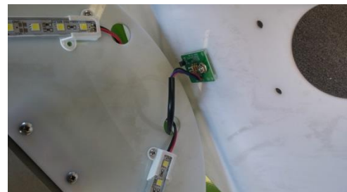
Figure 3: Laying the white backplate over
